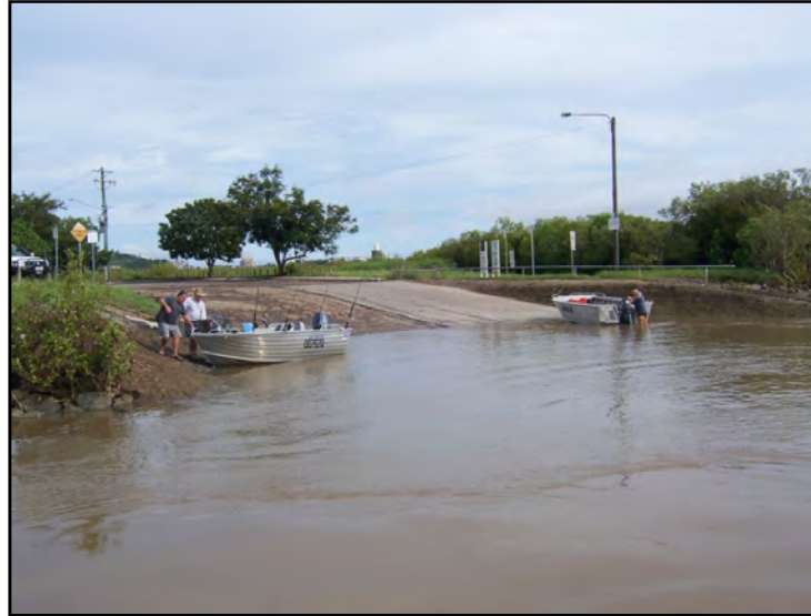
Figure 12. Boat ramp at Railway Estate.
