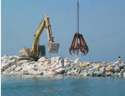
Excavator and grab barge placing rock offshore
