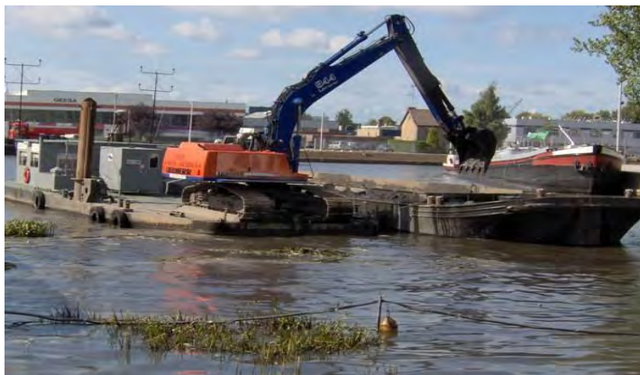
Figure 2 Typical backhoe dredge with split hopper barge being loaded
