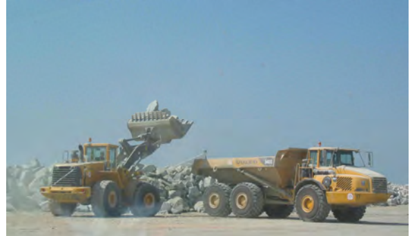
Loader rehandling armour to offroad dump truck
