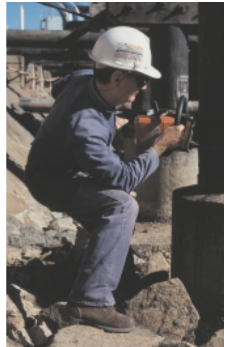
A TPA employee undertakes maintenance work under one of the berths.
