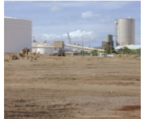
Construction began on Townsville Warehousing & Container Services' new facility in February 2001.
