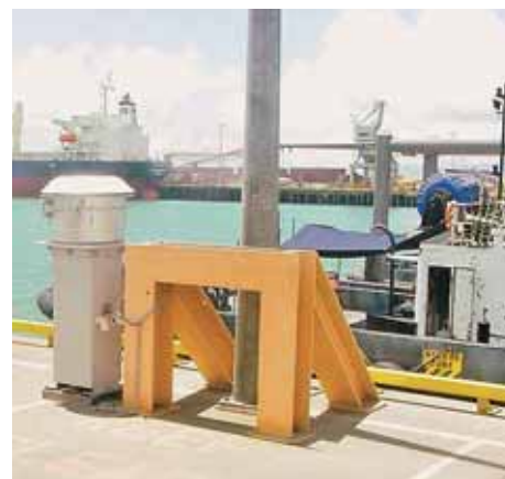
Figure 3. PM10 High Volume Air Sampler at Berth 9 with Berth 3 in the background.
